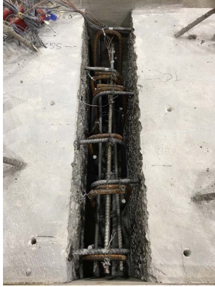
Figure 4-5 Innovative Joint on Specimen-4
